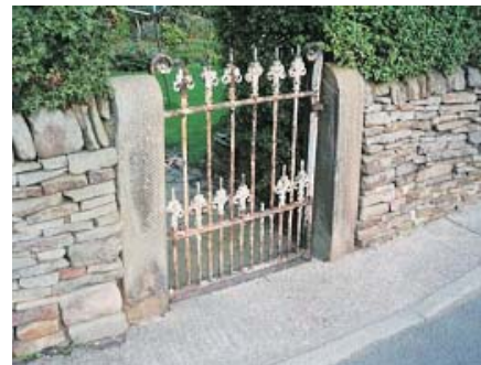
Stone gate piers and old gate – one of the small features that add to the character of the conservation area.
