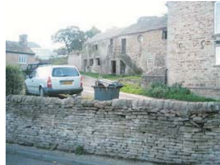
Typical stone wall. (Barns now demolished)
