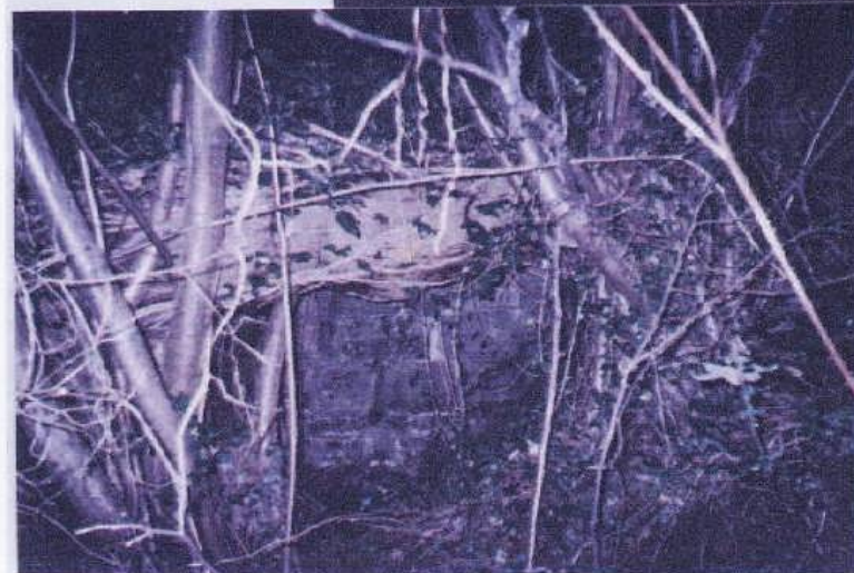
BLACKA DYKE BRIDGE
